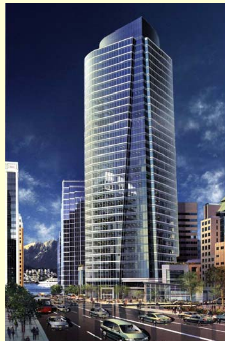
Bentall 5 once Phase II is completed
